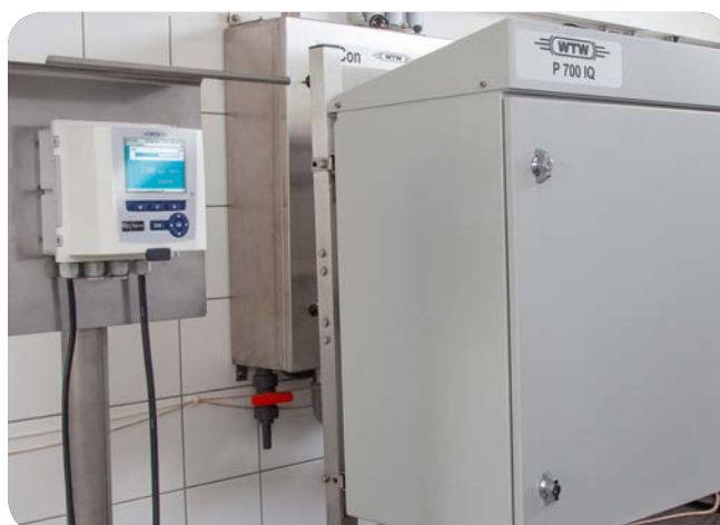
System 282/284 with Phosphate analyzer P 700 IQ
