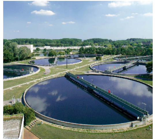
View over the Ludwigshafen wastewater treatment plant
