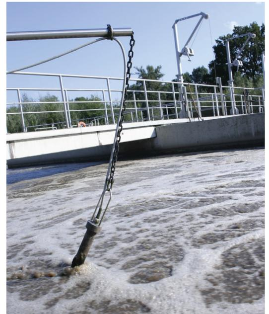
An IQ SENSOR NET dissolved oxygen sensor deployed directly in the aeration basin for continuous monitoring and control of aeration.
