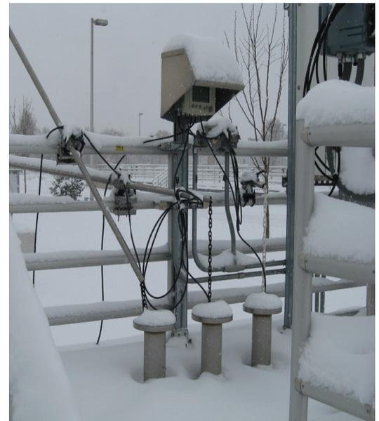
The IQ SENSOR NET 2020 XT terminal mounted tank side provides continuous process monitoring and control - even in harsh conditions.
