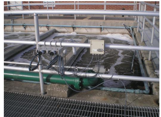
An IQ SENSOR NET module mounted tank side along with sensors for continuous process monitoring and control.
