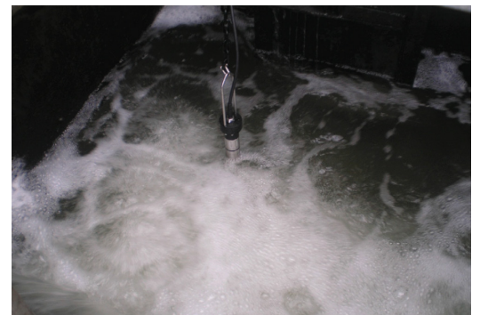
Figure 2: IQ SENSOR NET VARIION® sensor in Final Effluent
