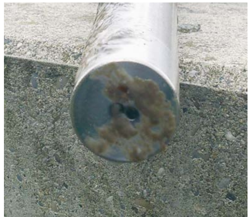
ViSolid® 700 IQ with switched-off cleaning system is completely covered with a biological layer after 16 days.
